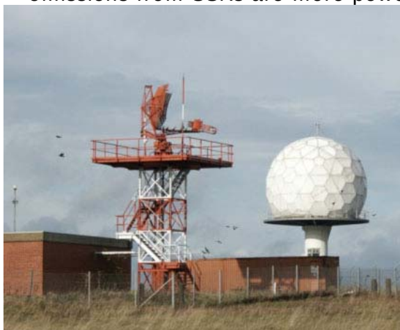
Figure 2-3: Secondary Radar (left) and Primary Radar (right)
